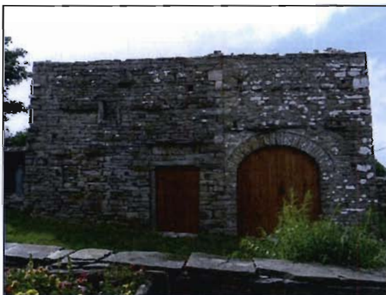
View of building from the east
