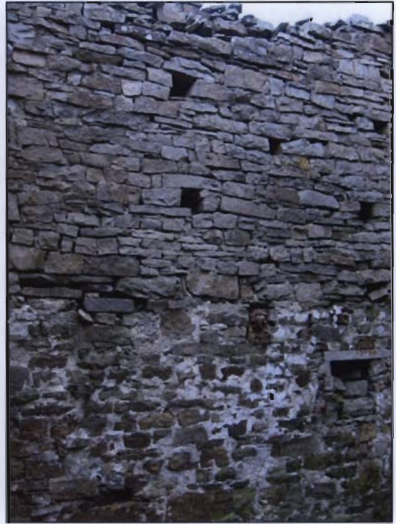
Typical interior wall, southern room
