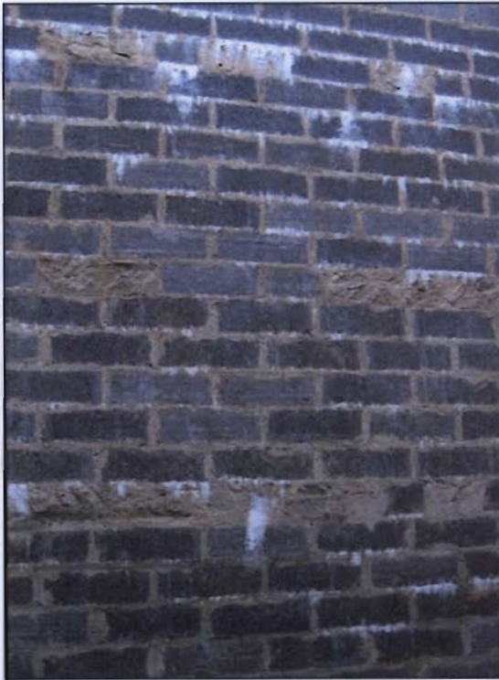
Interior wall, south end
