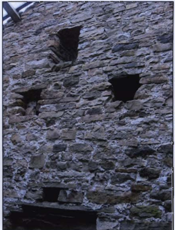
Typical interior wall, northern room
