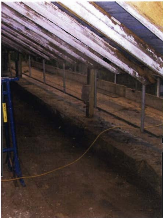
First floor opening with block infill removed
