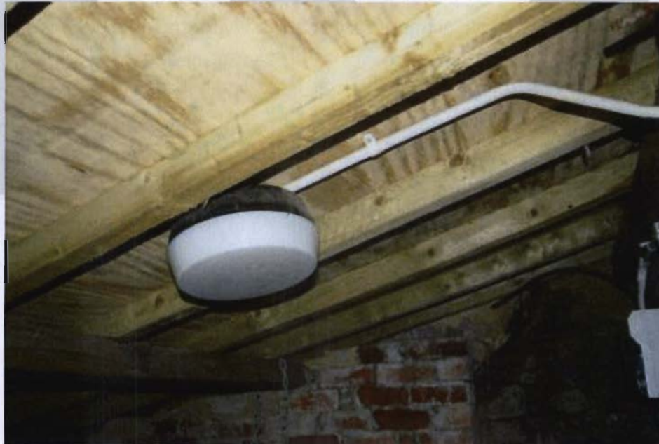
Underside of the roof to the outbuilding as existing
