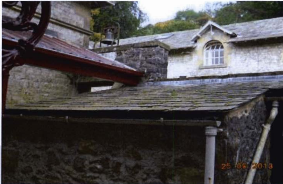
External roof covering as existing
