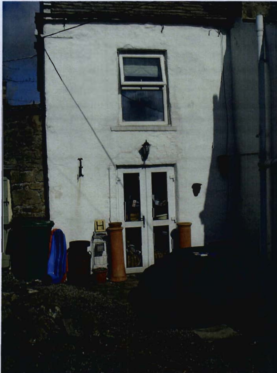
Rear view showing location of new 2 storey utility and bedroom extension
